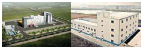
Flour mill plant under construction in Vietnam CJ Yihai Plant for Pre-Mix product in China
