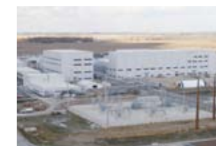
Production facilities in Iowa, USA under construction(Lysine)
